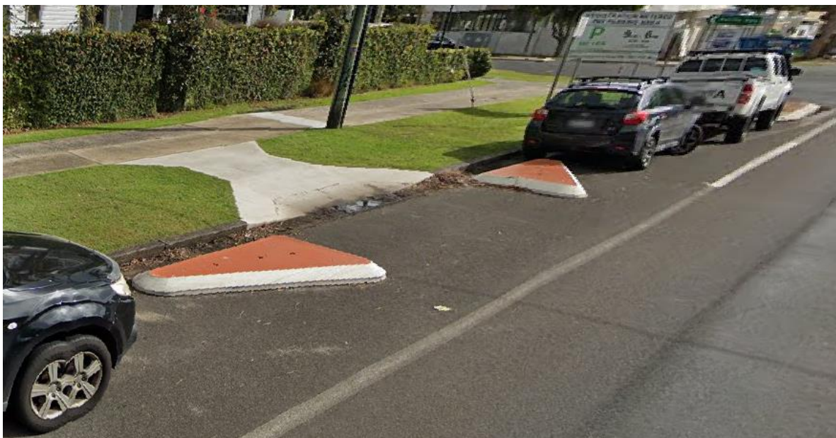
Figure 5: Example of Pedestrian Build-Out (Kerb Extension)
