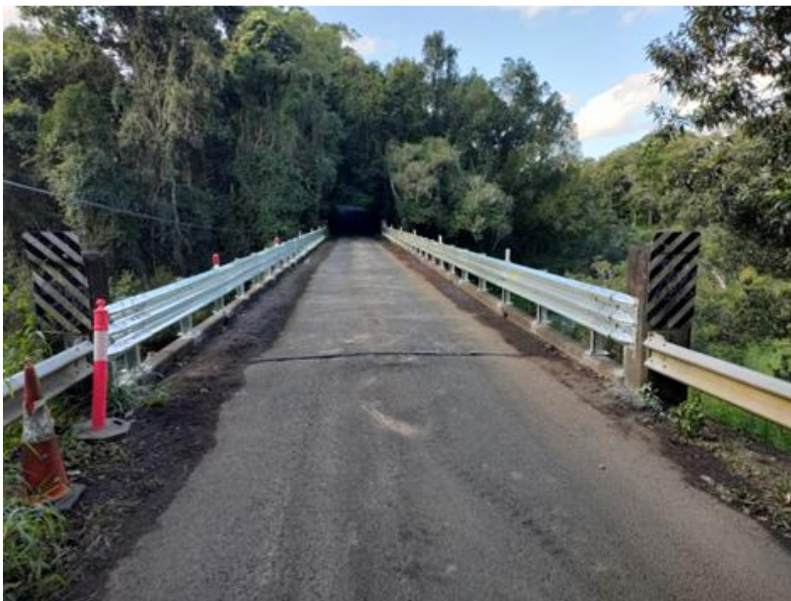
Keyes Bridge Guardrail replacement
