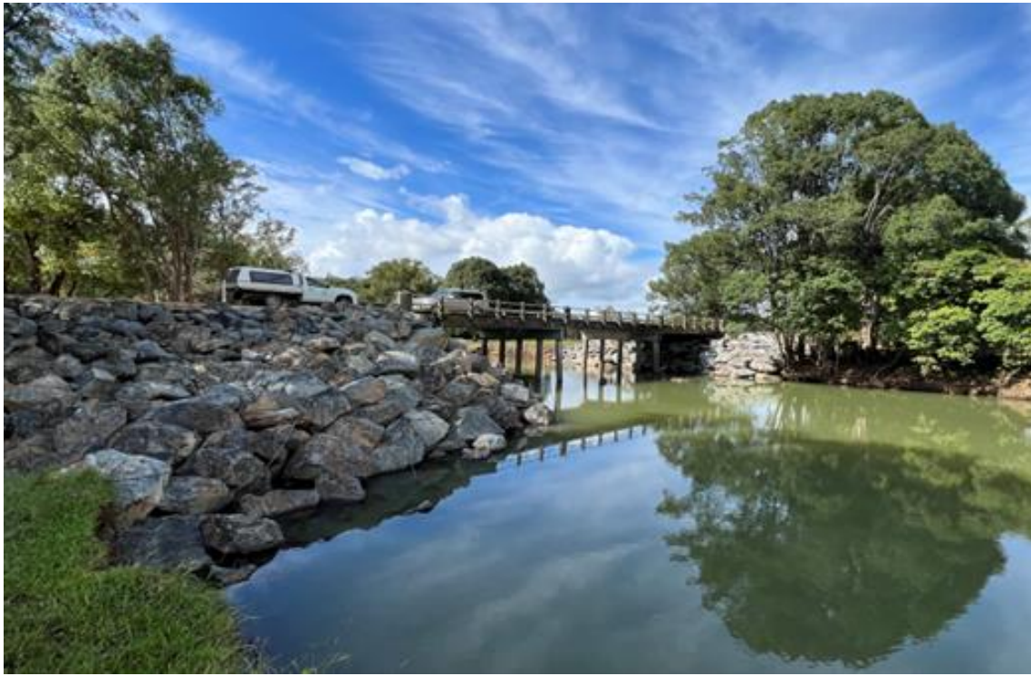
Williams Bridge (Main Arm Road) after abutment replacement
