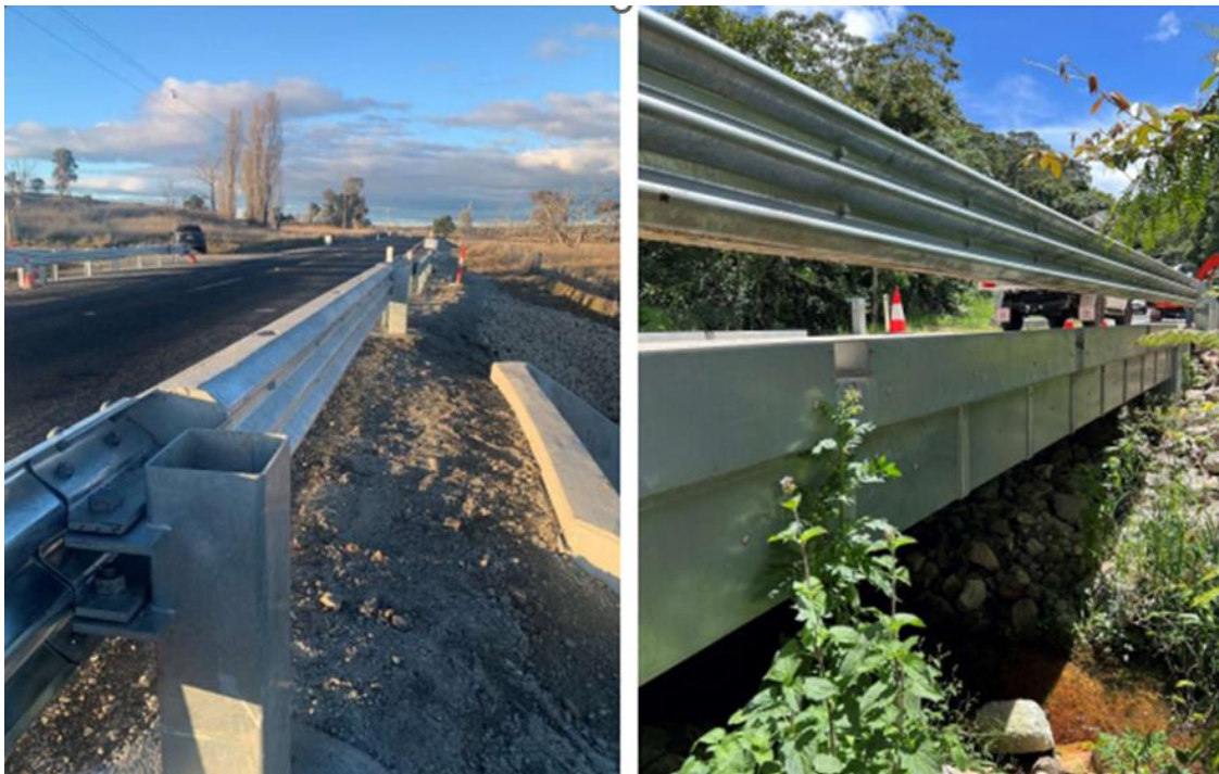
Croc Guard Guardrail proposed for Jubilee Avenue, Mullumbimby
