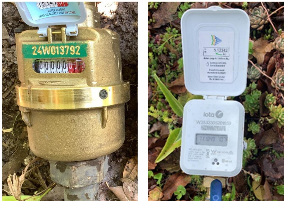
Figure 1 – A typical analogue water meter used in Byron Shire (left) and a digital water meter used during Council's DWM pilot project (Right).
