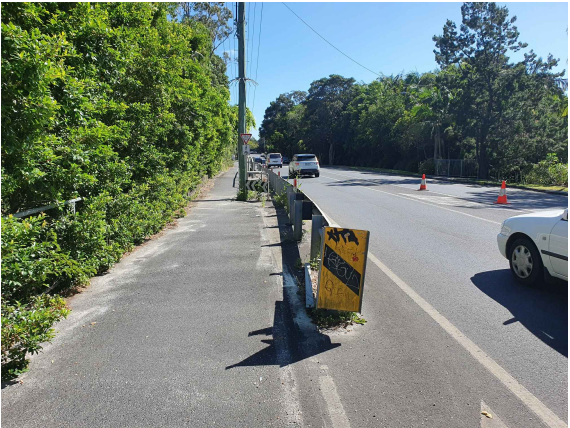
SITE PHOTO - EXISTING GUARD RAIL (LOOKING NORTH) NOTE: PROPOSED TO MAINTAIN EXISTING ASPHALT CYCLEWAY AND INSTALL PRECAST KERB AS PER IMAGE BELOW TO DELINEATE VEHICLE TRAVEL PATH BUT NOT INHIBIT STORMWATER FLOWS TO THE OPEN CHANNEL SYSTEM.
