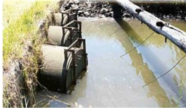
Figure 4: An example of a closed floodgate. This image was sourced from the NSW Department of Primary Industries.
