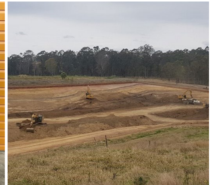
Landfill cell 4c due for completion in 2023
