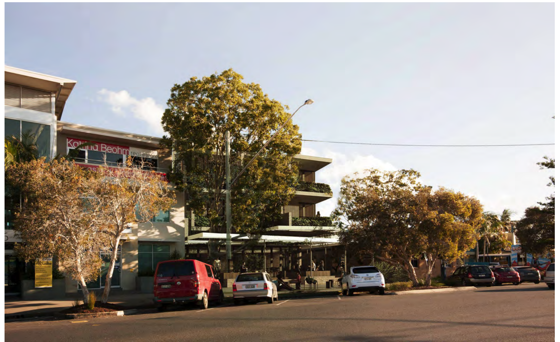
NORTH EAST PHOTOMONTAGE: The form is shrouded by established trees, with only a corner protruding from the canopy, this was the intended design.
