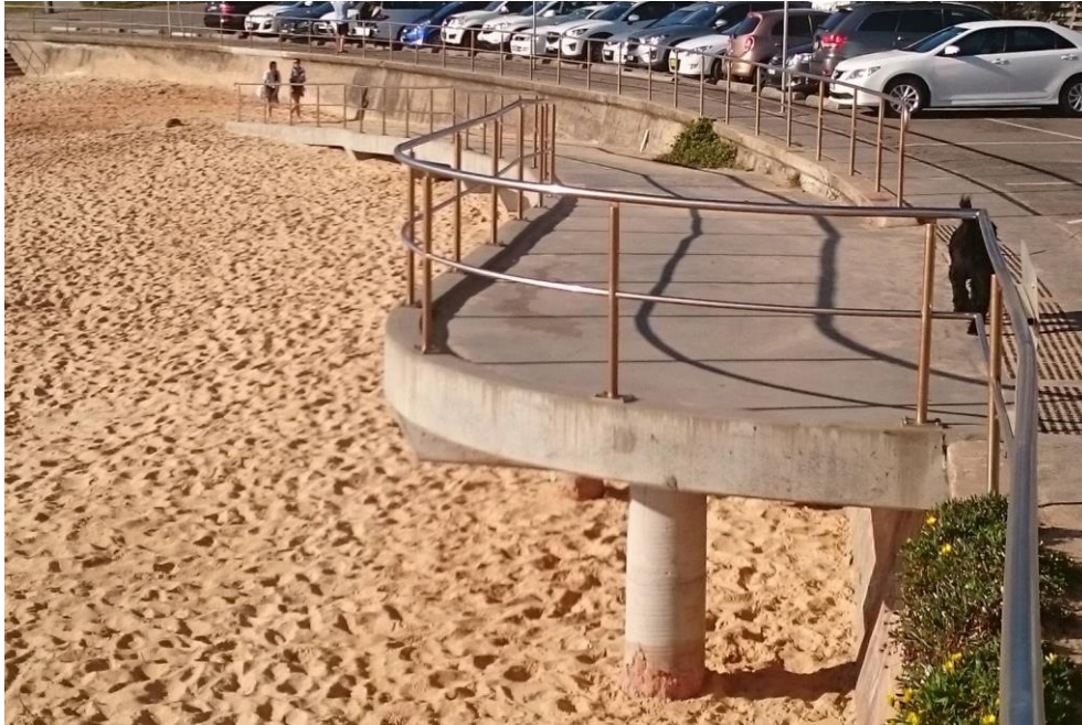
Figure 10. Reinforced concrete ramp at Curl Curl
