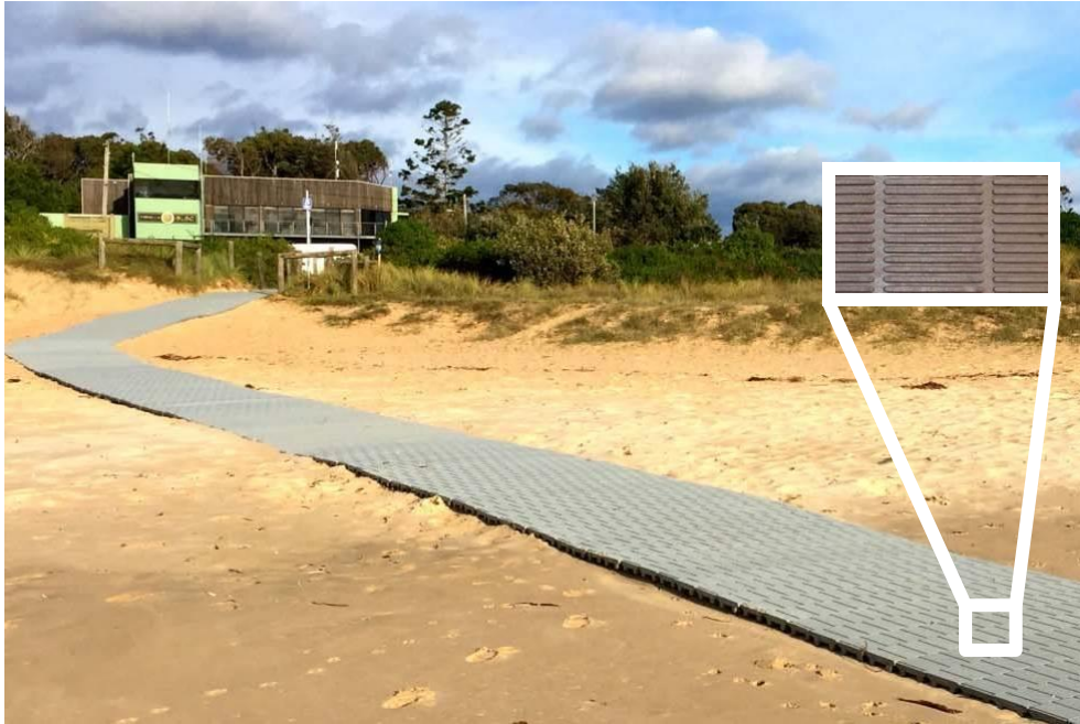
Figure 7. Modular plastic ramp at Pambula Beach (source: Replas)
