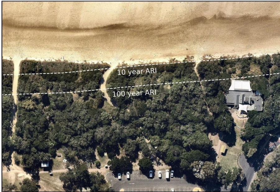
Figure 4. Approximate storm erosion hazard lines (image: Nearmap)
