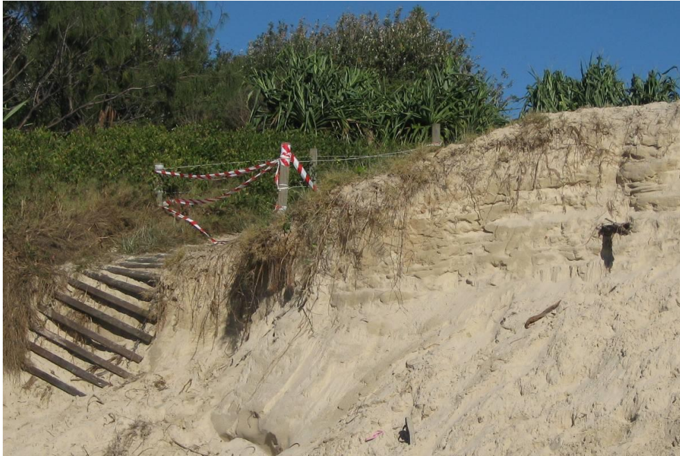
Figure 6. Destabilisation of board and chain path after dune erosion (source: J Carley, WRL)
