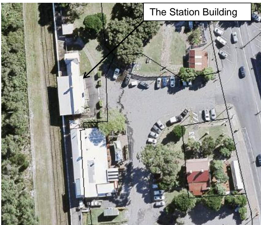
Figure 3: Location of Station Building
