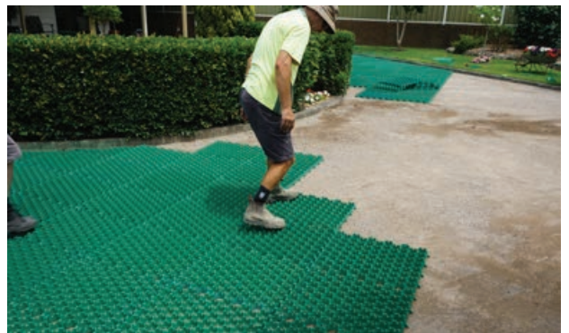
Laying out Econogrid 40 porous pavers
