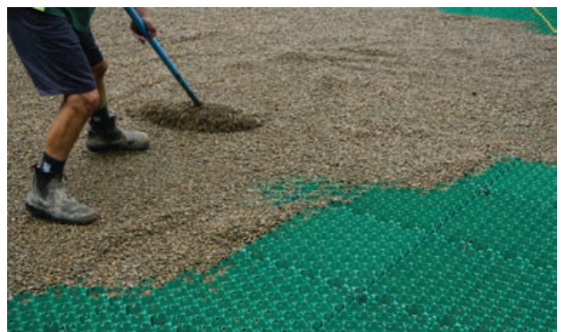
Filling pavers with Nepean River Bed Stone
