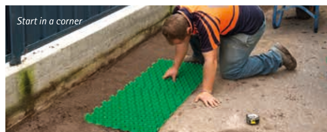
Pavers can be cut to fit
