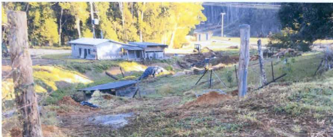
Picture B (below) No silt traps.
