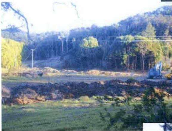
Picture 5. Filling First Order watercourse October 2016.
