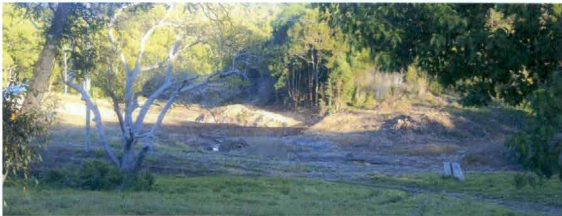
Picture B (below) No silt traps.
