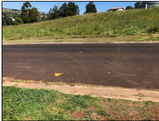
Existing fire hydrants in Rankin Drive.
