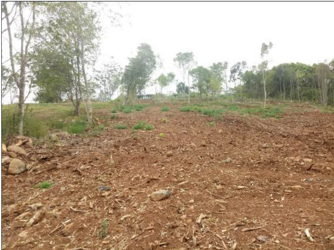
Photo 3 - View west and upslope across subject site.
