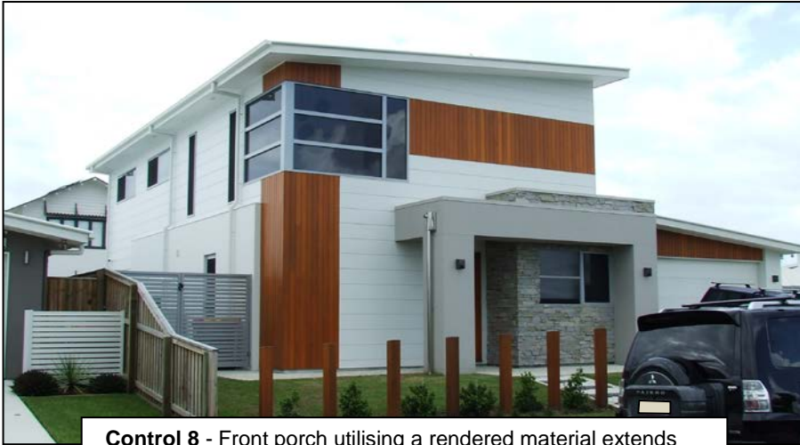
Control 8 - Front porch utilising a rendered material extends into front articulation zone. Control 13 - Open front fence delineates property boundary but allows street surveillance.
