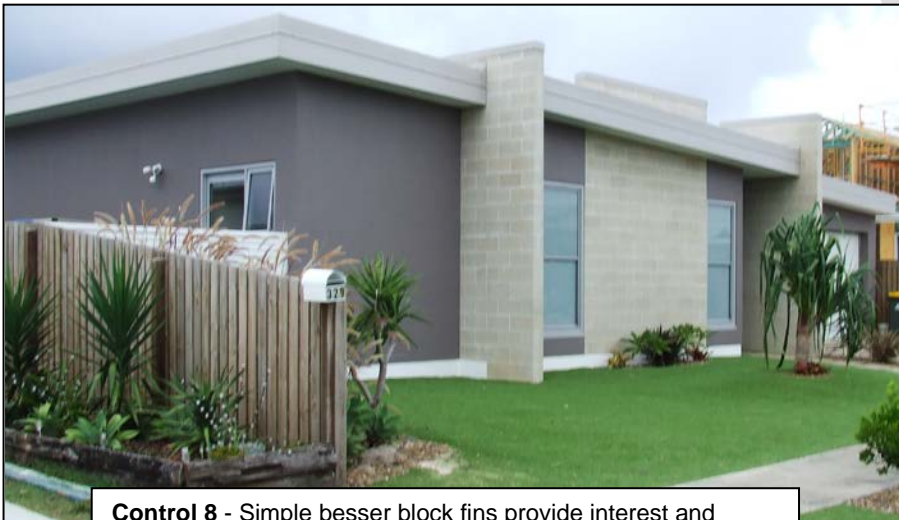
Control 8 - Simple besser block fins provide interest and variation to the front elevation extending into articulation zone.
