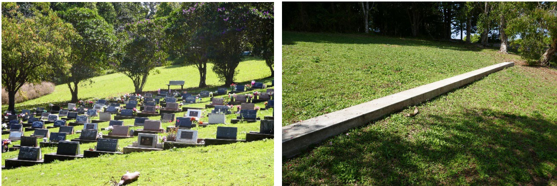
Figure 14... Old stepped beams and the new one.
