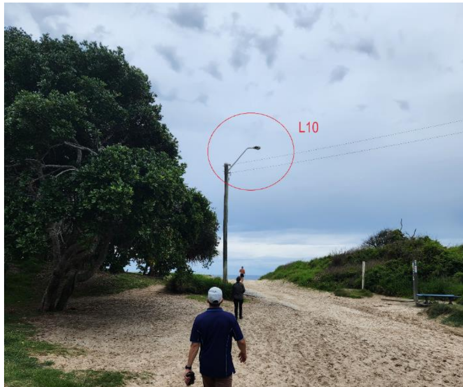
Plate 9: Essential Energy light fixture (L10) at highest point on the dunes, visible from the beach at New Jetty Park, Childe Street, Belongil.
