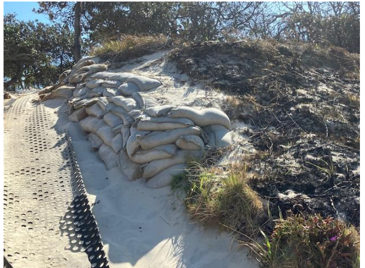
Photo 8: RHS of track – new sandbags installed (date unknown)
