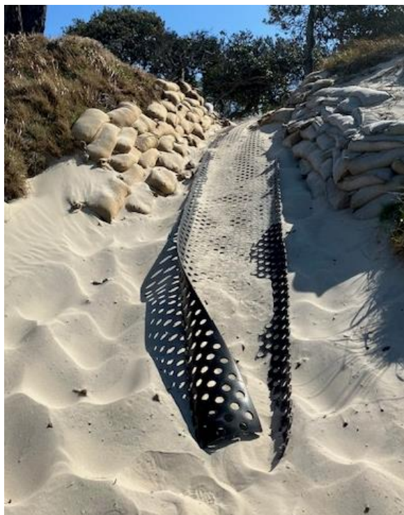
Photo 14: Seaward track matting visible (23/10/23)
