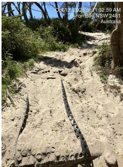
Photo 13: Landward access track plastic matting (edges peeling up)
