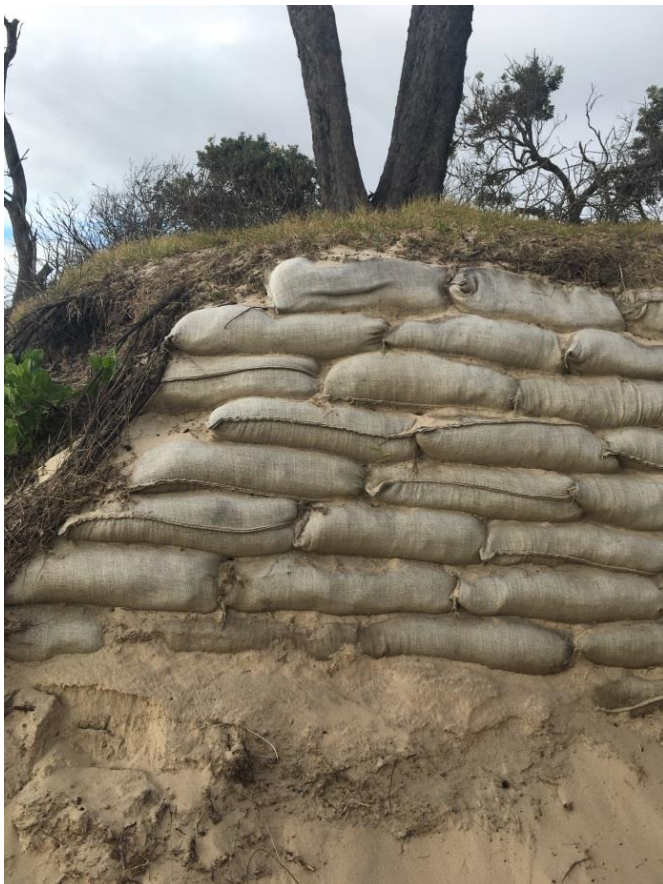
Photo 5: LHS of track – sandbags exposed (21/06/18)
