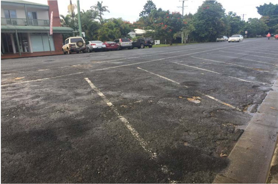
Figure 10: Poor road surfacing, Stuart Street
