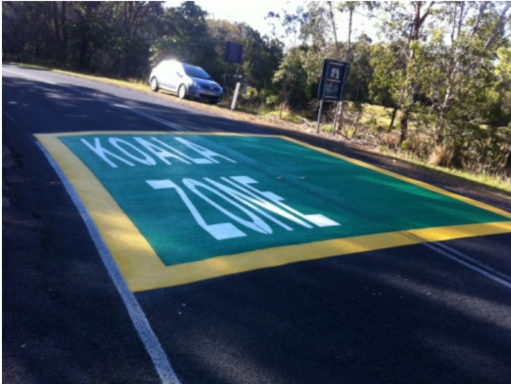
Plate H.1 Pavement treatment at Clothiers Creek Road (Source: Tweed Shire Council)
