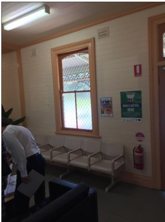
Figure 73: Original timber Sliding sash window.
