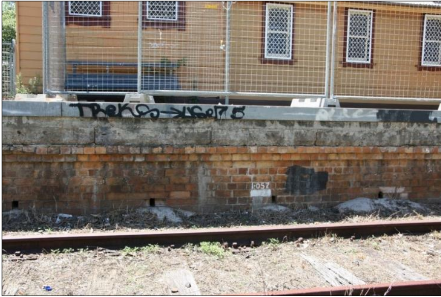
Figure 113: Detail of platform edge showing brick wall set beneath concrete slabs and topped with metal trim. Weir Phillips
