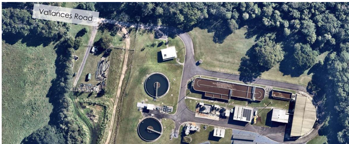
Figure 3-10 Current Aerial View of BVSTP.
