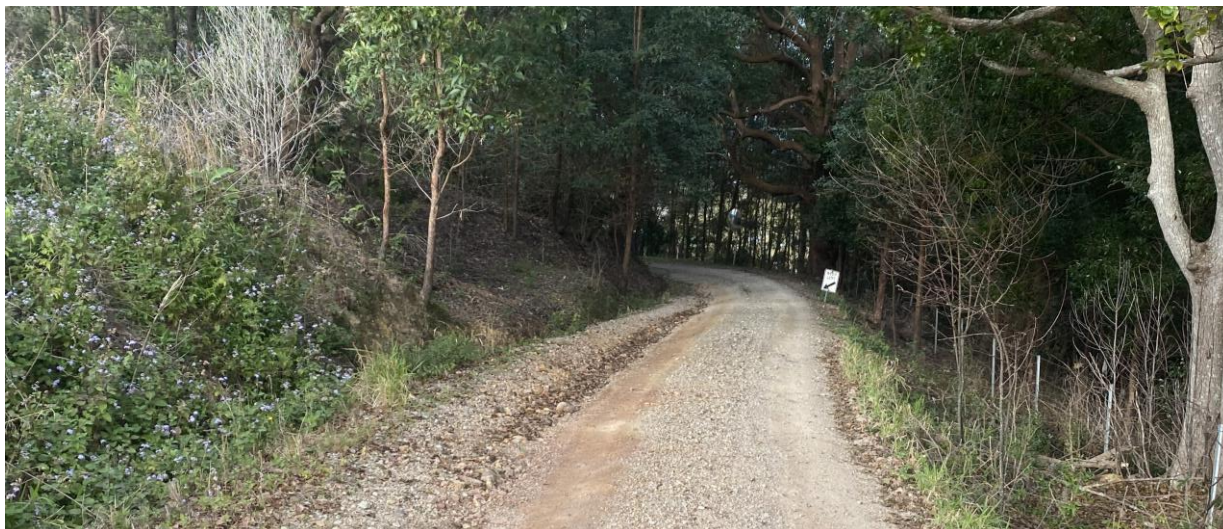
Figure 3-5 Typical Section of Old Nursery Access Road at Blind Corner.
