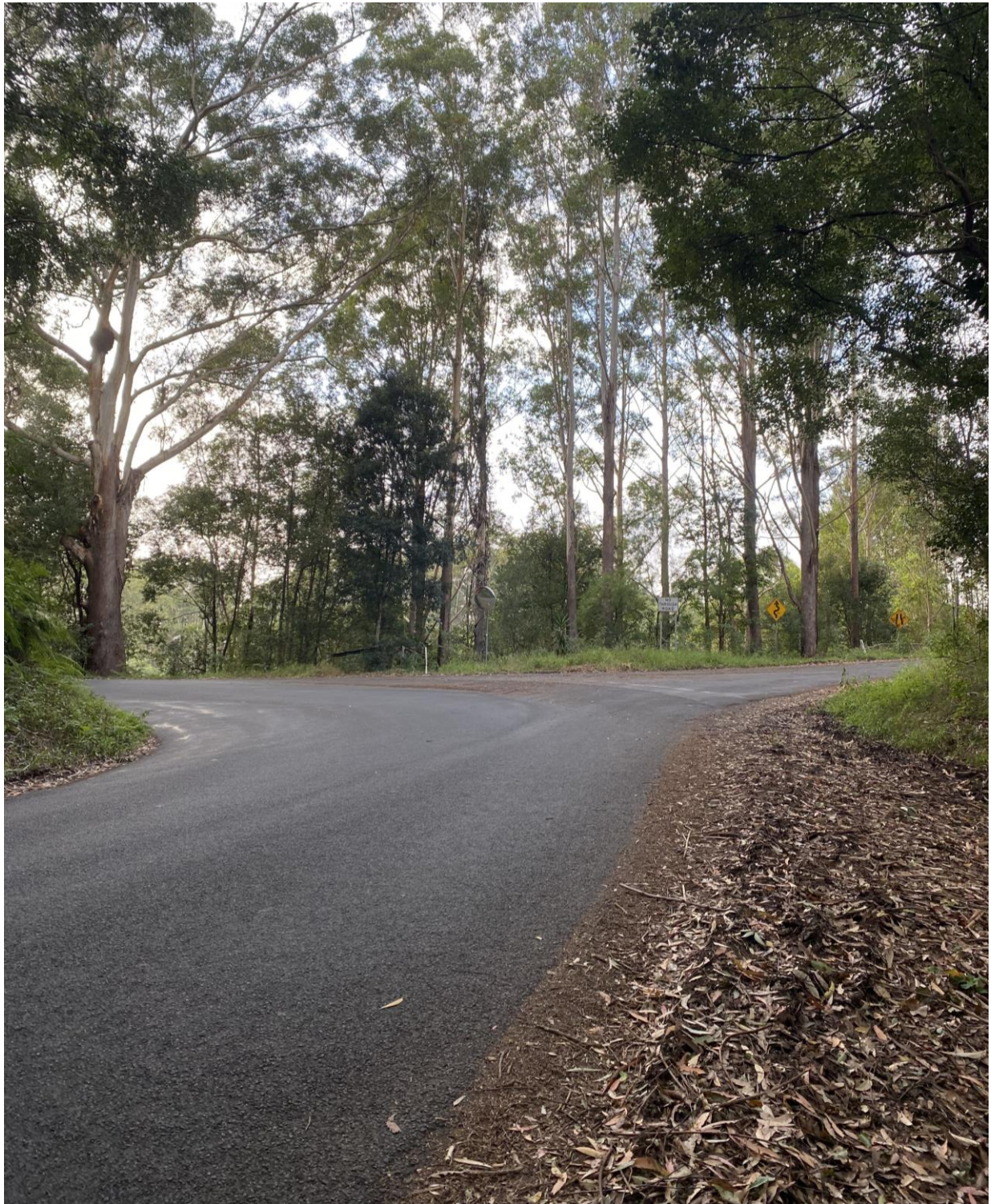
Figure 3-7 Coolamon Scenic Drive / Vallances Road Intersection – from Coolamon Scenic Drive, showing poor site distances for entrance into Vallances Road.
