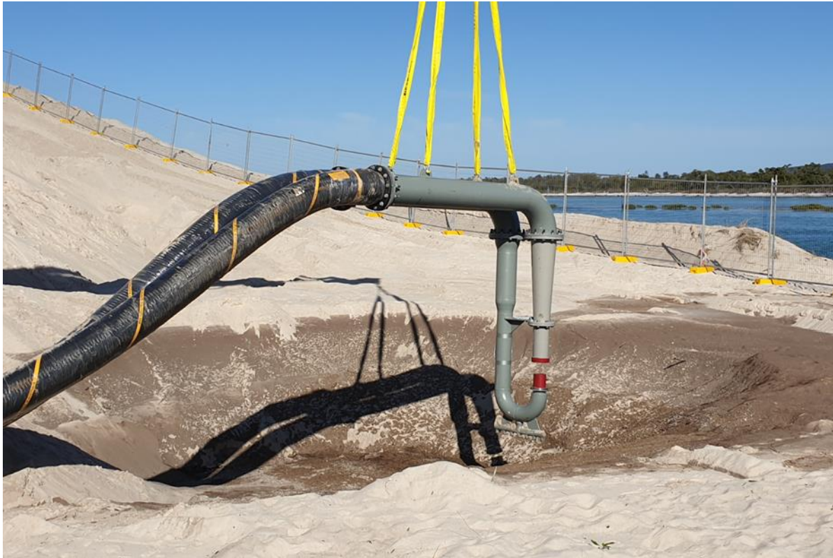
Figure 7: Photo of a jet pump being installed at Jimmies Beach.
