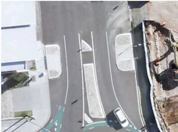
Figure 5-9 Pedestrian crossing facility with kerb extensions on Jonson Street, Byron Bay
