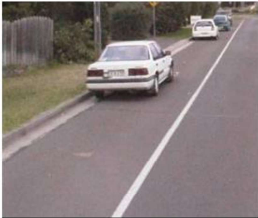
Figure 5-1 Edge line adjacent to moving lane
