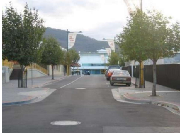
Figure 5-10 Pedestrian crossing facility with kerb extensions in Glenorchy, Tasmania
