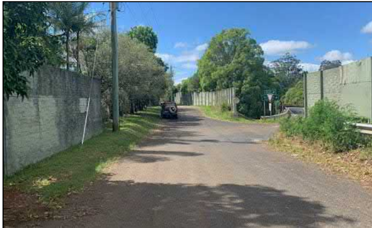
Granuaille Crescent looking south to Hinterland Way intersection
