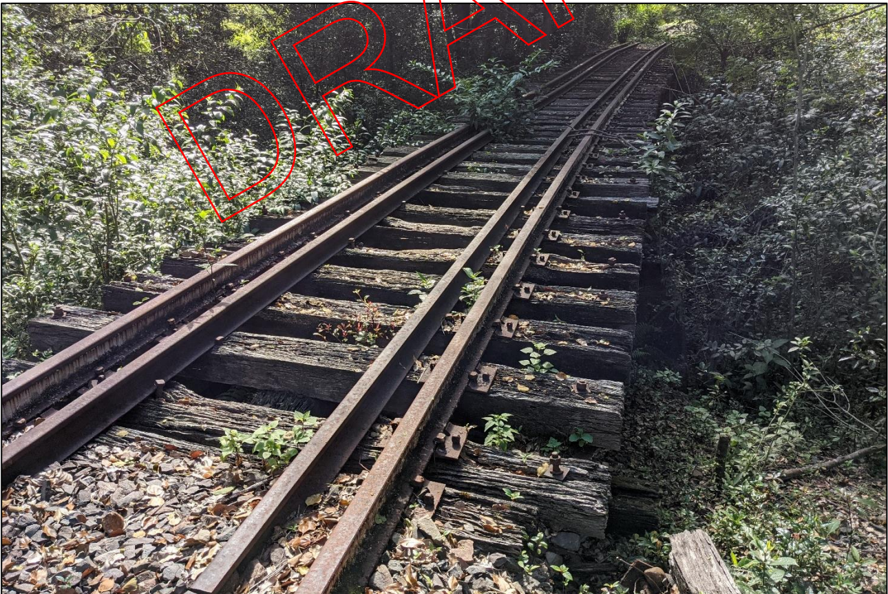
Figure 2.2 Timber Railway Bridge (Bridge 2)
