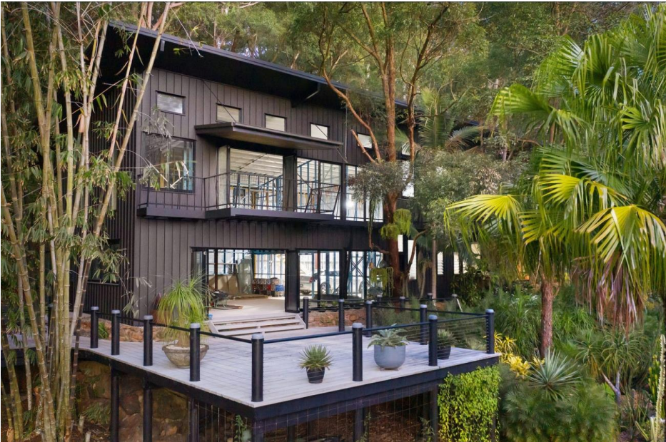
Upper floor balcony and deck and lower floor deck on Northwest Elevation
