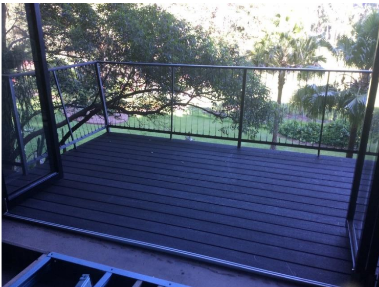
First floor balcony
