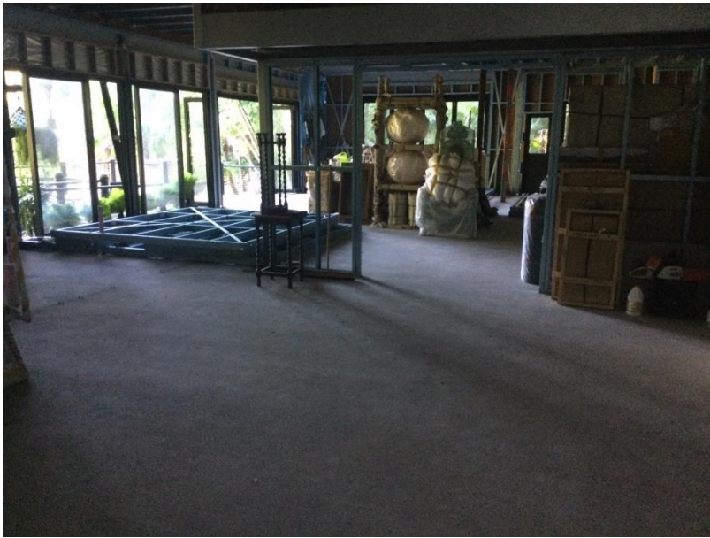
Ground floor area as constructed.
