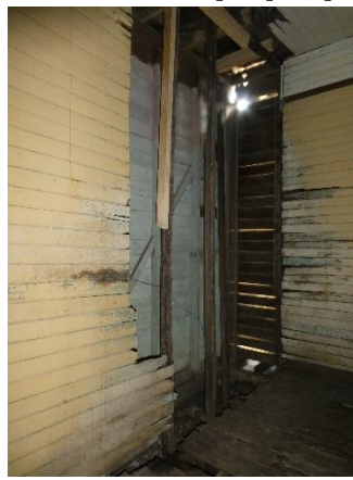
Southern side of bedroom wall behind frame.
