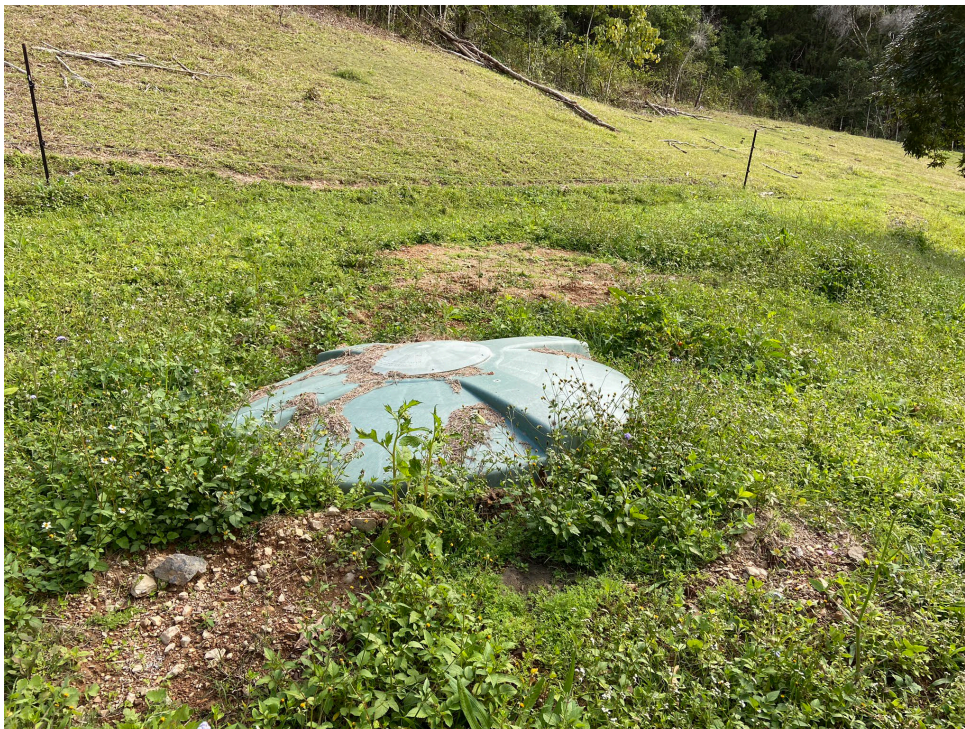
Photo D OSMS for Farm Shed
