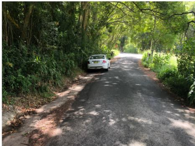
Plate 2 – 3m Sealed Section Settlement Road (view towards Main Arm Road Intersection)
