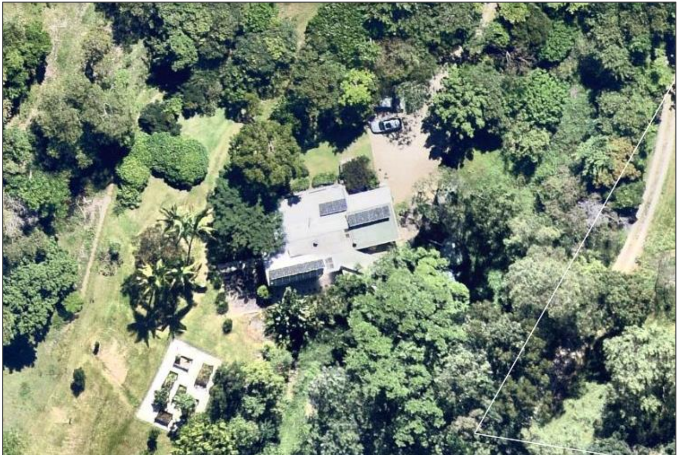
Figure 2: Existing unauthorised dwelling
