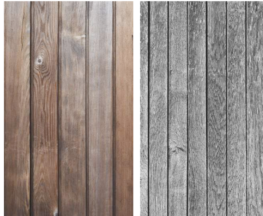
T -VERTICAL TIMBER CLADDING
