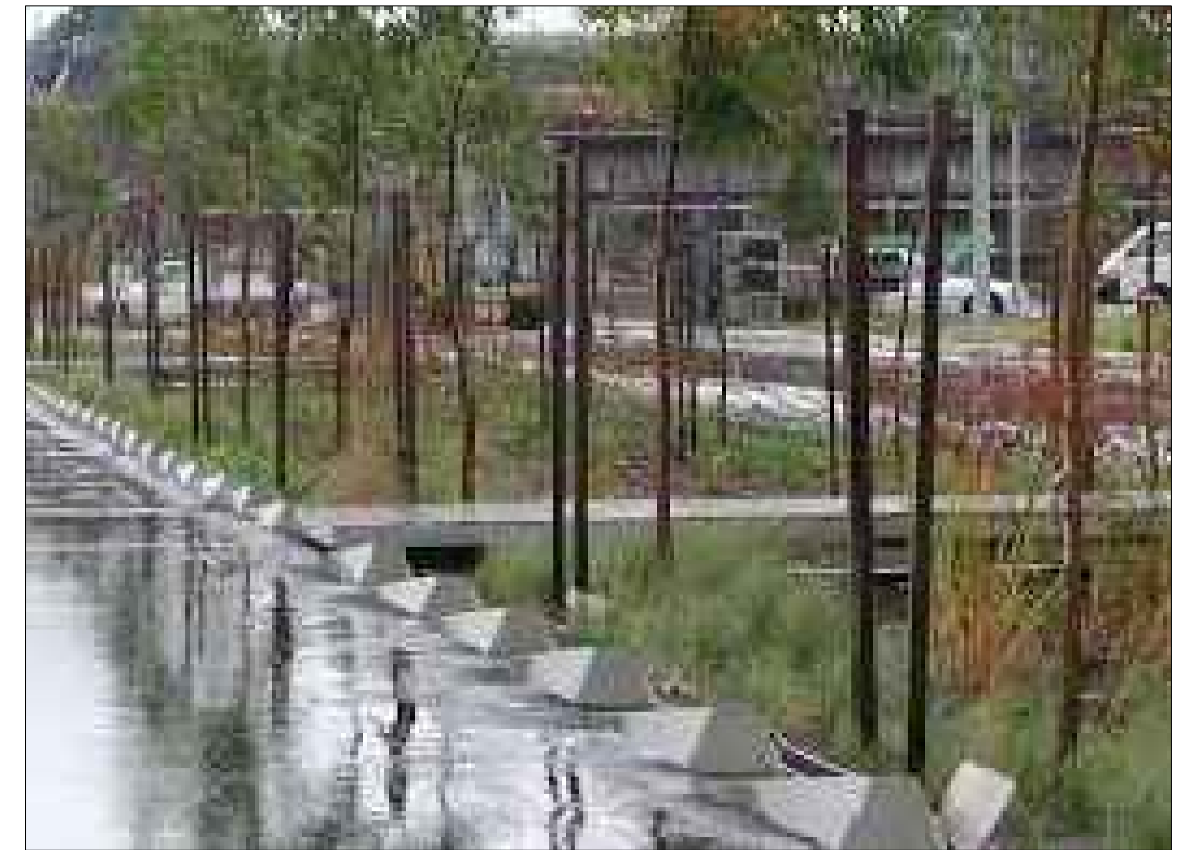
VEGETATED RAINGARDEN INCLUDING KERB BREAK
