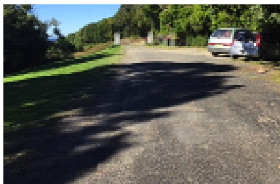
Figure 5 End of Council Maintained Section
