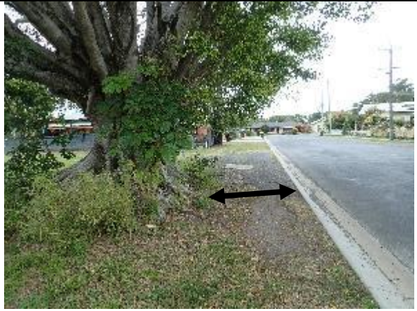
Figure 11: Approximately 2m from edge of buttress to kerb. Highly compacted area
