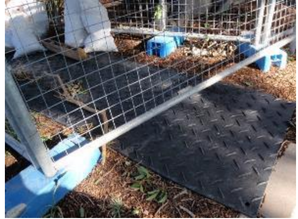
Image 6: Good – Load sharing device over mulch
