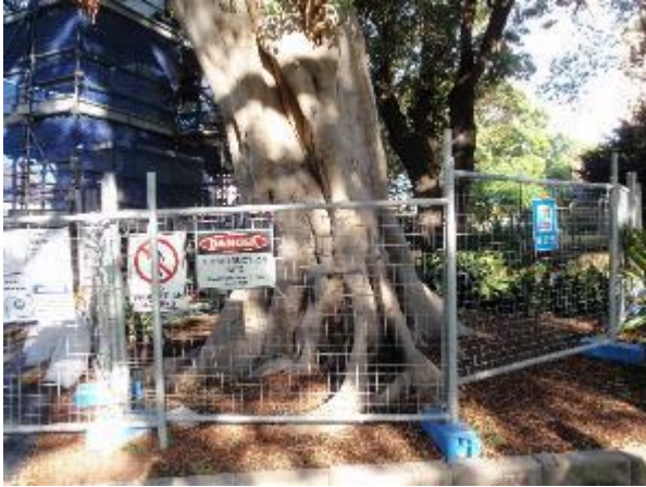
Image 1: Good – Fencing and mulch
