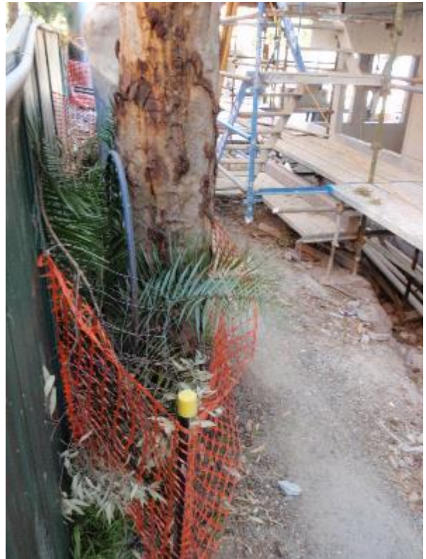
Image 4: Bad – Compaction due to no mulch or load sharing device over a high traffic area; with minimal tree protection
