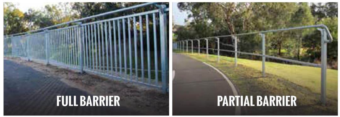
SHARED PATH BARRIER FENCE EXAMPLES
