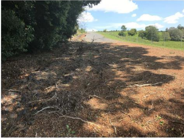
Alstonville - Site 1 – Looking West.
