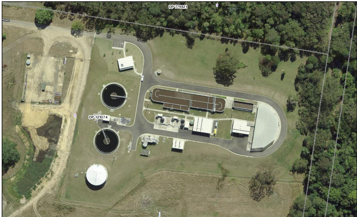
Figure 6 – Existing Sewage Treatment Plant
